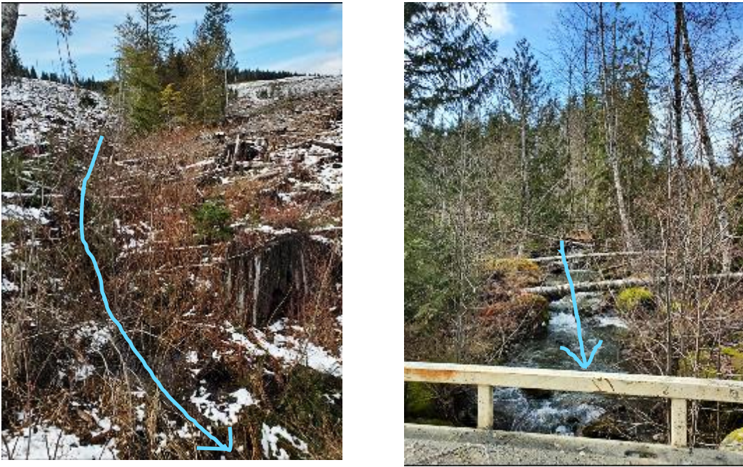
Figure 4: Ground verified Riparian Disturbance identified (the blue arrows trace the stream channel)
