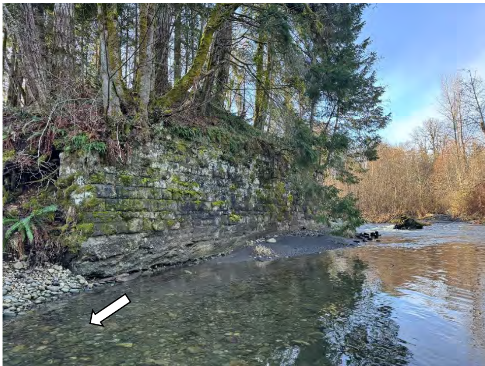
Photo 2. Concrete footings of historic railway bridge. Arrow indicates flow direction. Photograph collected March 6, 2025.
