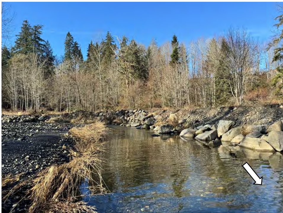
Photo 6. Placed riprap along the river-left side channel. Arrow indicates flow direction. Photograph collected March 6, 2025.
